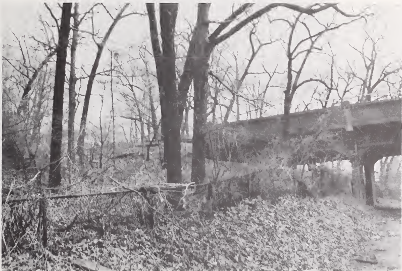
11. Forest Park Drive Overpass
